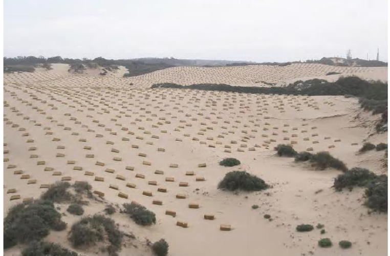
Straw bales deployed as dust mitigation measures
